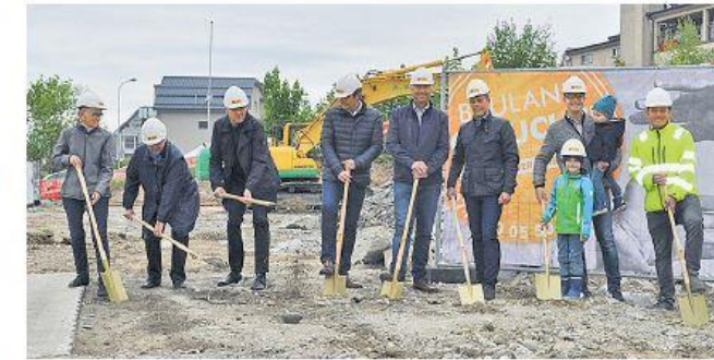
Baustart in Staad (CH).
